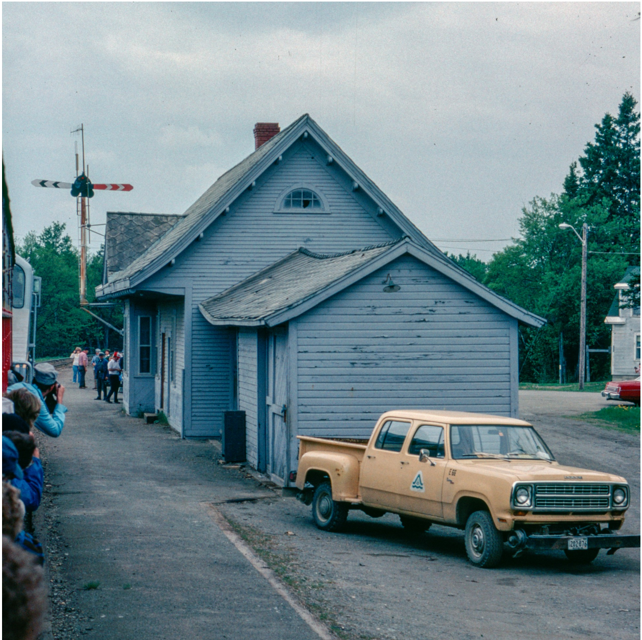
Richard B. "Dick" Gassett shot this picture of Oakfield Station on June 1 st , 1980, from an excursion train. JoeyKelleyPhoto.com Collection
