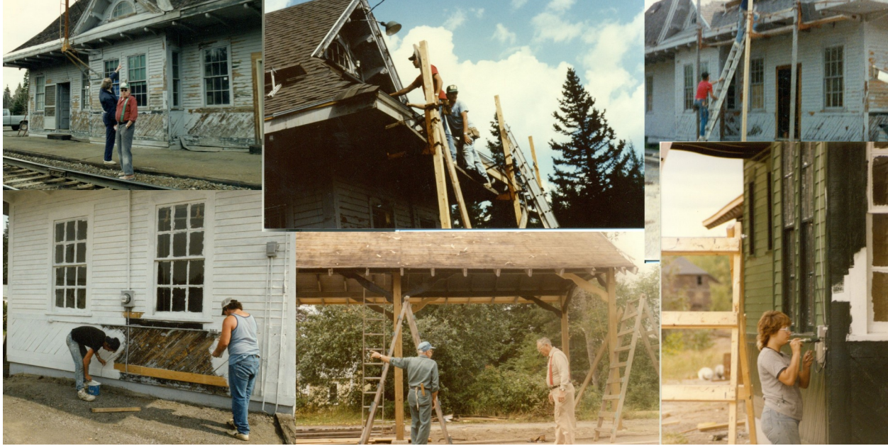
Volunteers Get it done! Station Restoration photos from the collection of the Oakfield Historical Society
